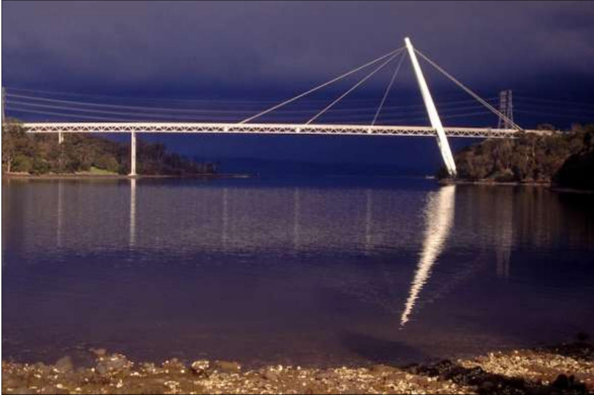
Batman Bridge — Norton Harvey
