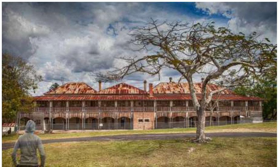
5. Found Outside the Walls
