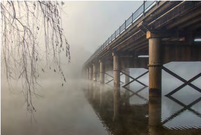
Windsor Bridge 1874-2020 APS Merit Paul Evans
