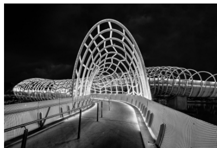
Webb Bridge Acceptance Andrew Leach
