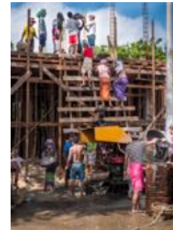
Construction site Myanmar Acceptance Peter Roupas
