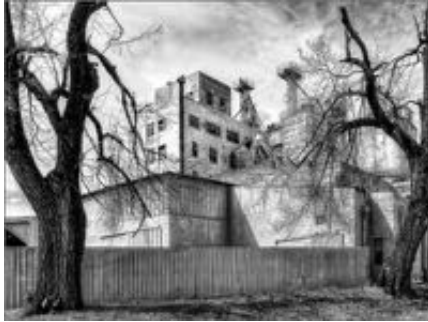
Derelicts guarding derelicts Acceptance Jan Lee EPSA FPSA
