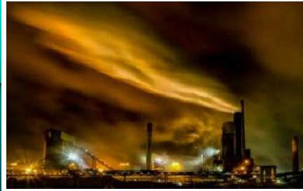
Port Kembla Cokeworks 5a Acceptance Rob Oyston
